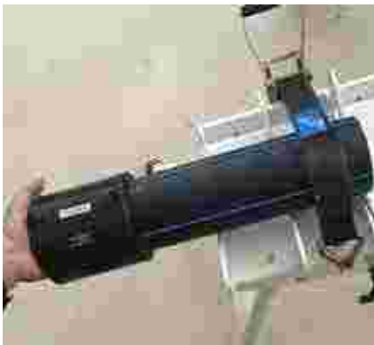
4- Insert pipe into electrofusion coupler.
